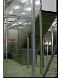
The Mecanova vertical shower scald incorporates insulated doors for maintenance, as well as exterior and interior stairs for easy access for maintenance and cleaning. To facilitate daily cleaning work, the scalding system incorporates interior lighting.
